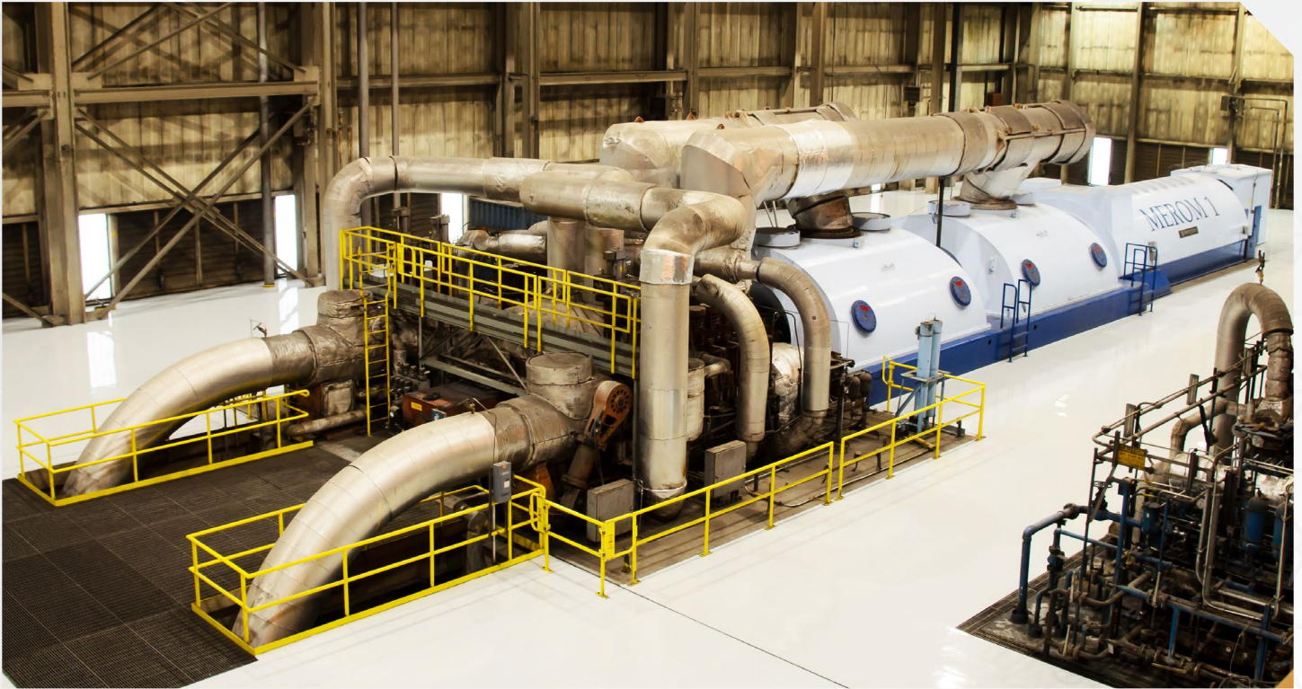
Merom Generating Station in Sullivan County
