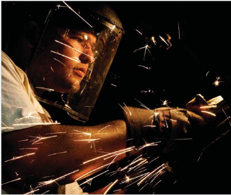
A welder fixes a break in one of the turbines at Ratts during outage maintenance.
