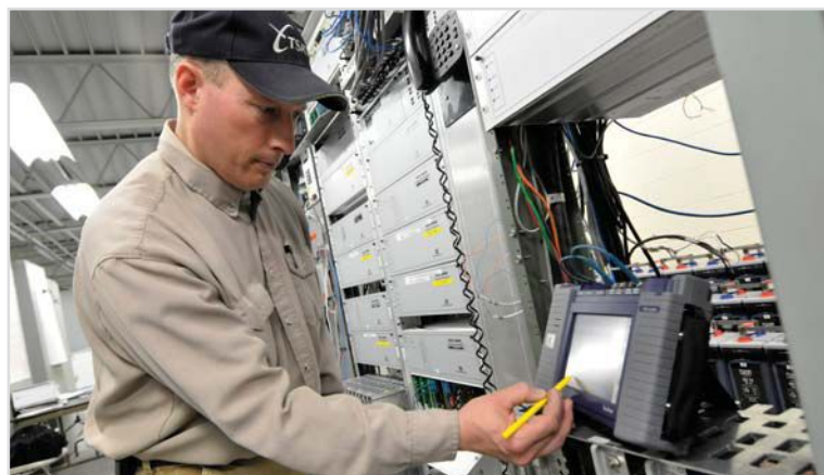
Hoosier Energy Communications Technician Bryan Abel tests digital communications circuits. Diagnostic tools help detect potential problems in the field.
