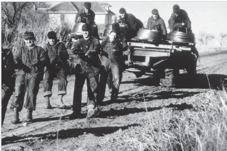
Stringing distribution line by hand was a primitive and time-consuming method, but it got the job done.
