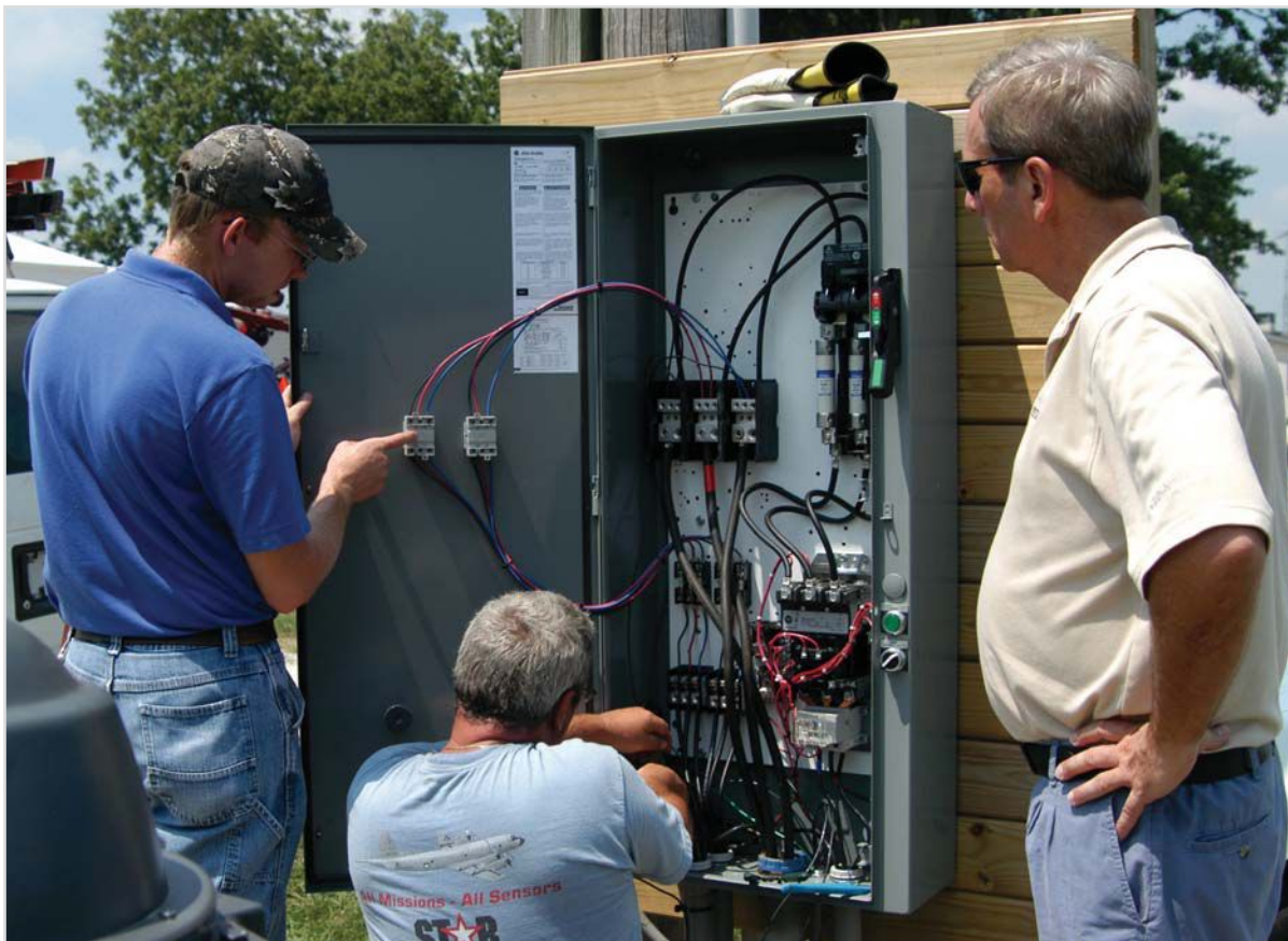
Energy efficiency specialists set up a load control device to help a farmer in Bartholomew County match field irrigation times with off-peak billing rates.
