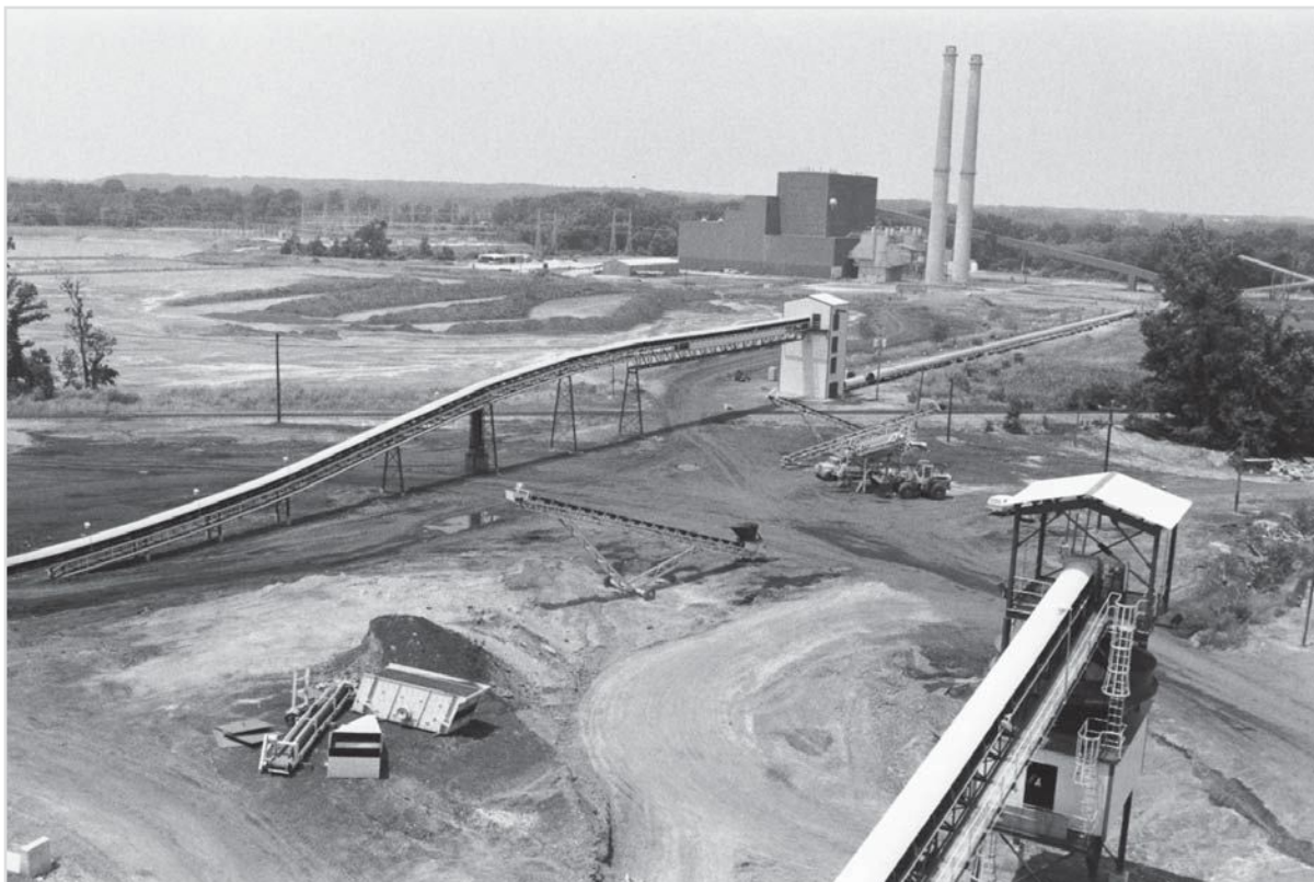
The Ratts Station utilized the abundant coal resources of southwestern Indiana. The conveyor in the foreground carries coal from the Solar Sources wash plant to the station.
