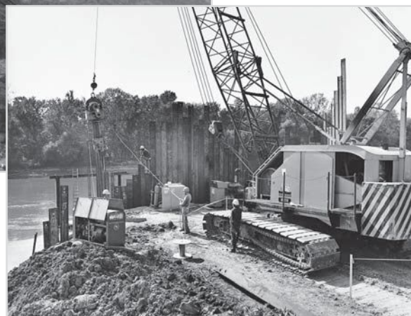
Construction crews built a cofferdam on the Wabash River as part of the construction of the Merom Station's cooling system.
