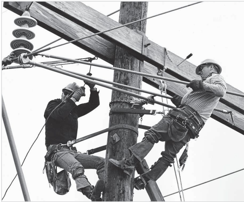
Hoosier Energy line specialists have long maintained the cooperative's transmission system. Bill Dunn and Howard Goss perform hot stick work on a transmission line in the mid-1980s.
