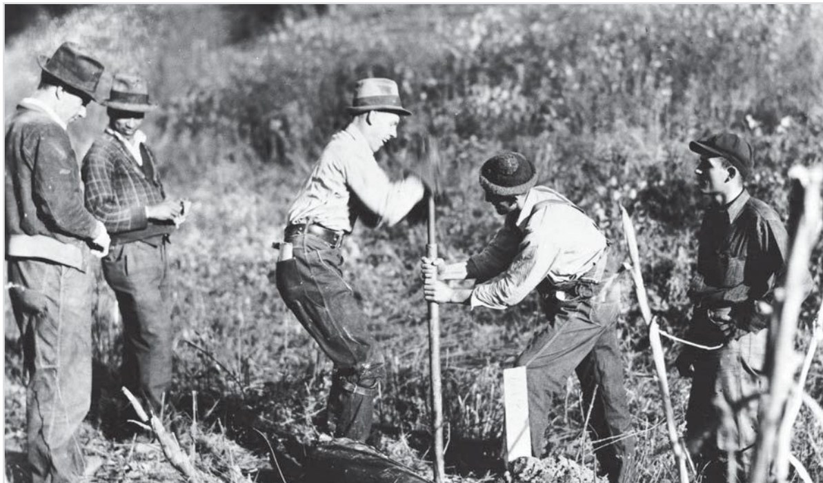
Distribution poles had to be cut, hauled and peeled before early rural electric cooperatives could string wire to farm houses.
