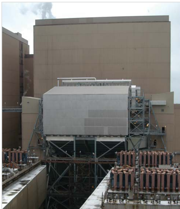
Selective catalytic reduction technology was instrumental in helping Hoosier Energy reduce air emissions 91 percent from 1983-2014.
